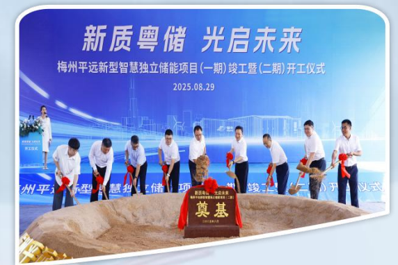
Commencement of the Meizhou Pingyuan (Phase II) Smart Energy Storage Power Station Project
